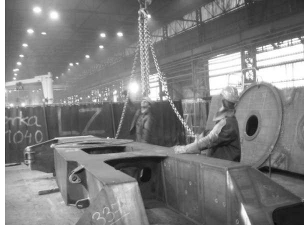
Fig. 12.4 The construction is placed on racks welding
