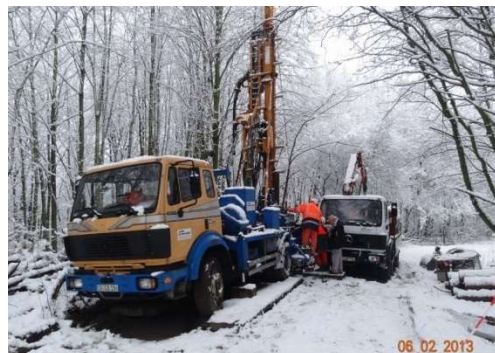
Fig. 17.11 Start of the research drill hole on the abandoned landfill
